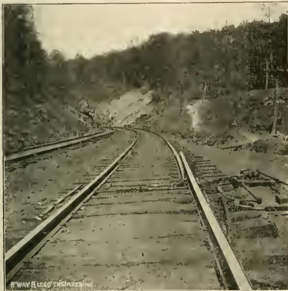
DERAILING SWITCH OPEN NEAR ENTRANCE TO OXFORD TUNNEL, D., L. & W. RAILROAD.
